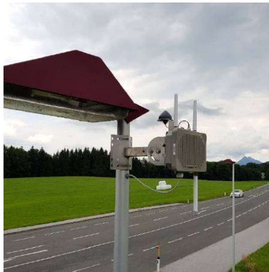
Figure 69: Kapsch TrafficCom RSU installed in Koppl (pilot site Salzburg): Location#5 (Source: Kapsch TrafficCom).
