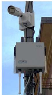
**Figure 34: Example of LINKS RSU with camera**
