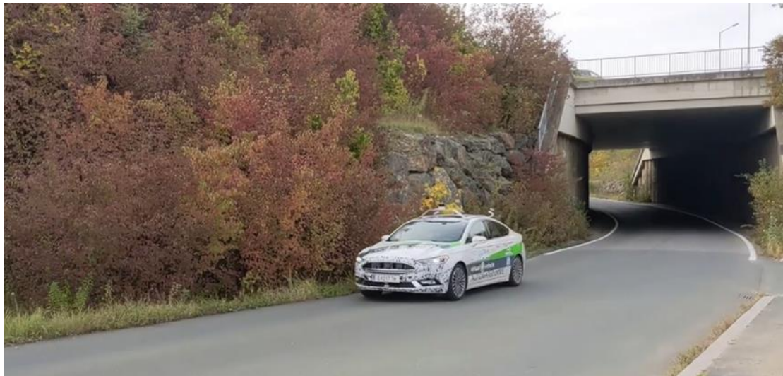
Figure 6: Segment B (dedicated road; front) and C (tunnel; behind). (Source: VIF)
