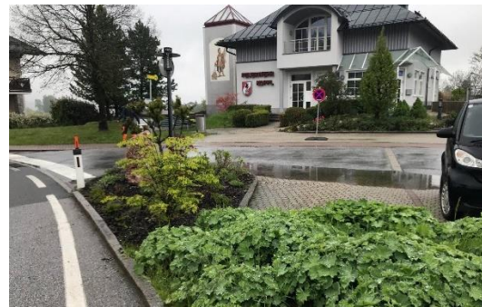
Figure 38: deep puddles at the stop "Koppl town centre" (Source: Salzburg Research)
